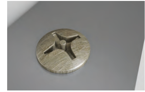
TAMPER RESISTANT HARDWARE All screws used on all the Behavioral Health units have been replaced with tamper resistant security screws.
